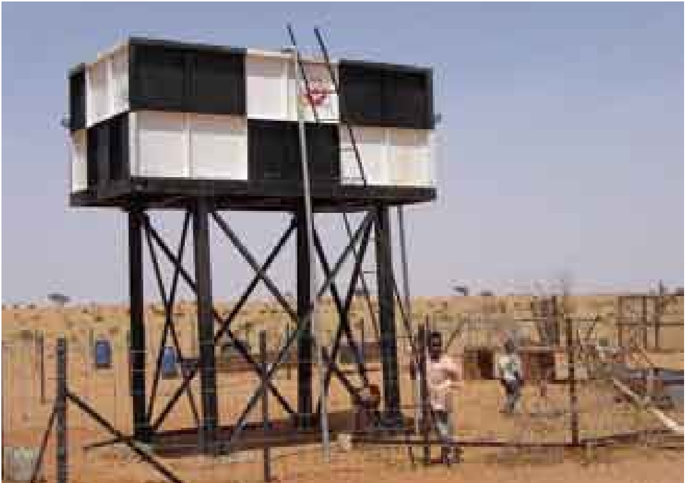
Storage facility made of mild steel, North Kordofan State
