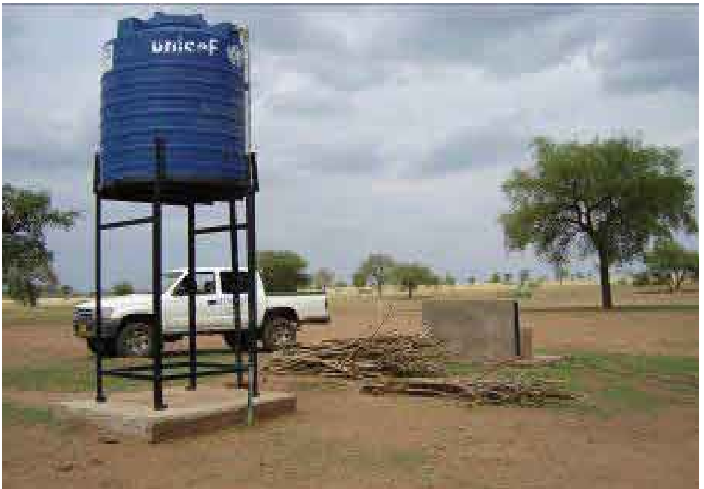
Small size storage facility in South Kordofan State made from PE material
